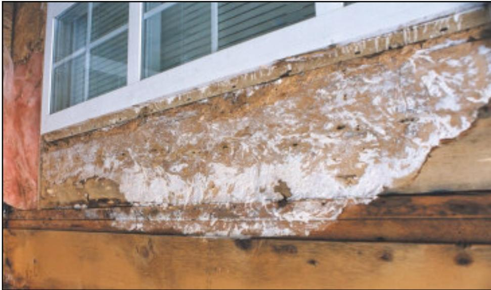
Wood-rotting fungi show typical fan-like growth of white mycelium. This fungus was spreading under exterior sheathing in a building which had faulty construction.
